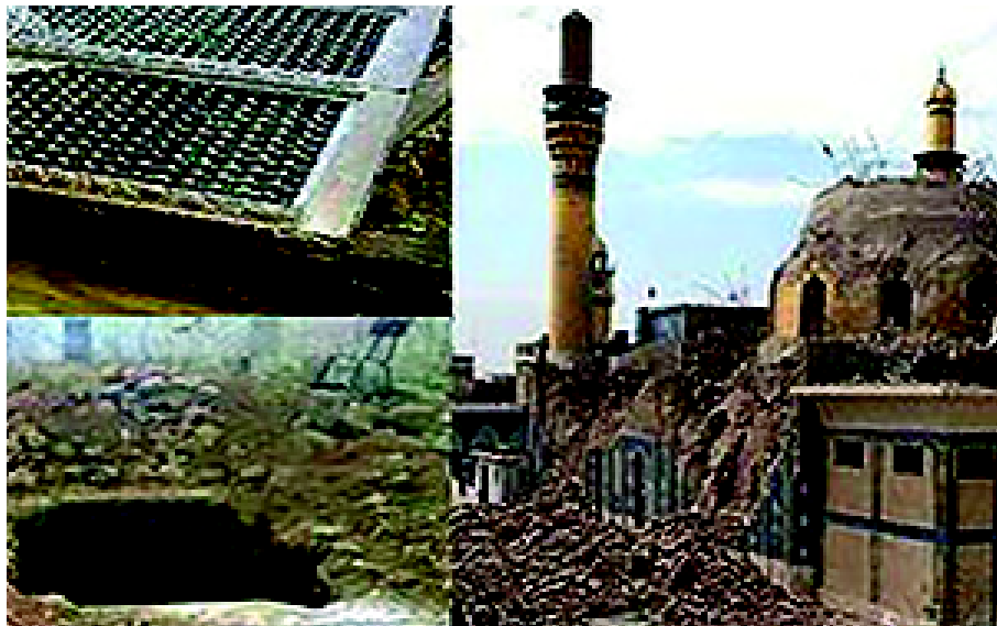
An sorrowful and painful image showing the vandalism and desecration of the shrine and the sand stone, which has attacked the shrine of Hjr bin Adi Al Kindi (may Allah's mercy be upon him) from inside and outside.
